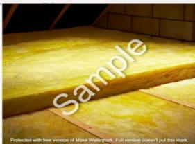
Insulation should be installed tight to the structure, without air gaps, and should extend to the wall insulation
