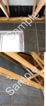
Eaves photograph should show loft insulation extending beyond the wall insulation to minimise cold bridging.
